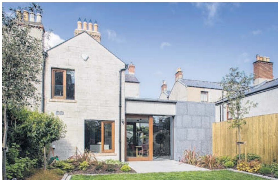
The redbrick front of the Victorian house in Rathgar, far left, and the rear extension in limestone, left and above, designed by Gottstein
